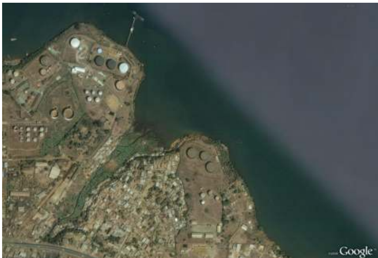
Plate 1.24: Google image of the Addax facility at Kissy Terminal.
