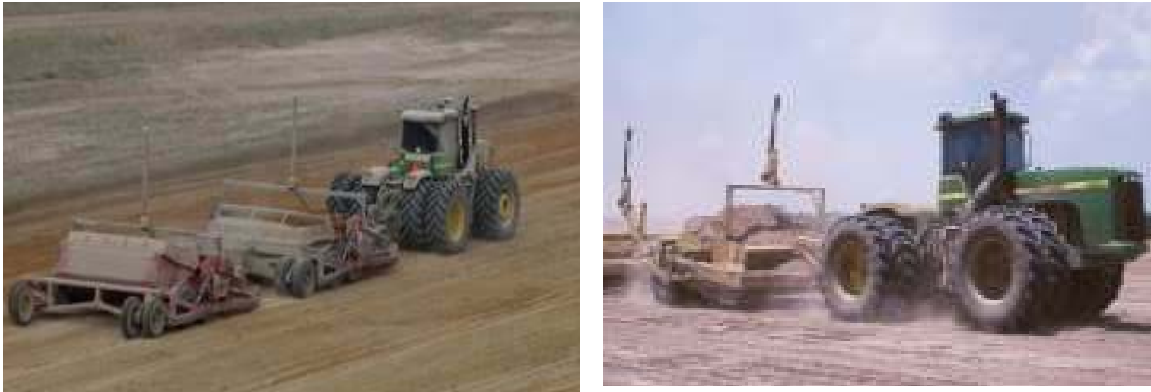
Plate 1.4: Laser controlled land forming equipment
