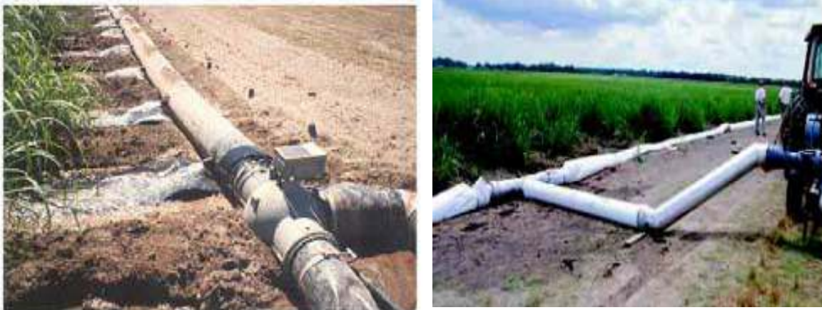
Plate 1.8: Surge valve controllers operating on layflat gated irrigation pipes
